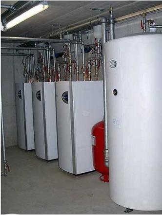
**Figure 2: One of the three technical rooms; you can see heat pumps and 750l buffer tank**
