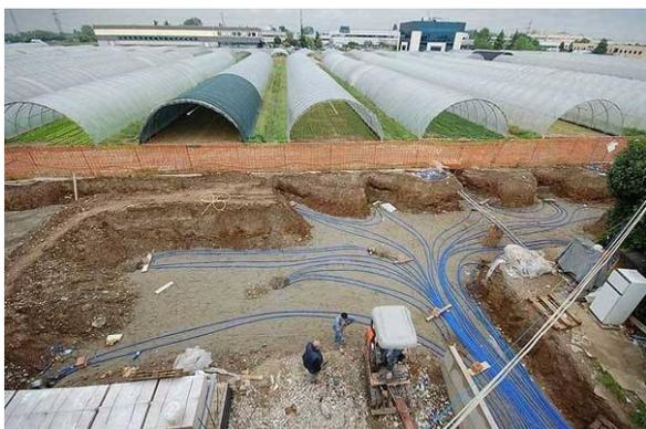
**Figure 3: one of the three closed boreholes fields (F1 building): the 4<sup>th</sup> from the left is the incorrect depth borehole n.47**
