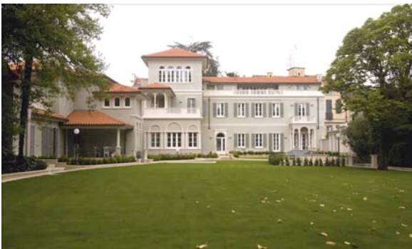
Figure 4: outside park of the building; vertical geothermal probes are installed under garages
