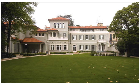
Figure 4: outside park of the building; vertical geothermal probes are installed under garages
