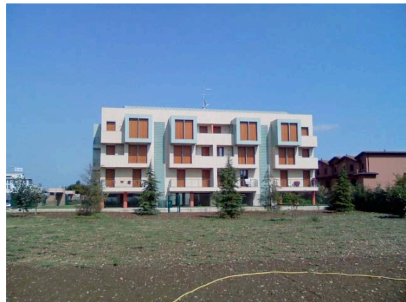
Figure 1: Front side of one of the three aligned residential buildings
