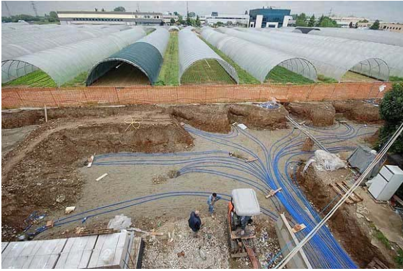
Figure 3: one of the three closed boreholes fields (F1 building): the 4 th from the left is the incorrect depth borehole n.47
